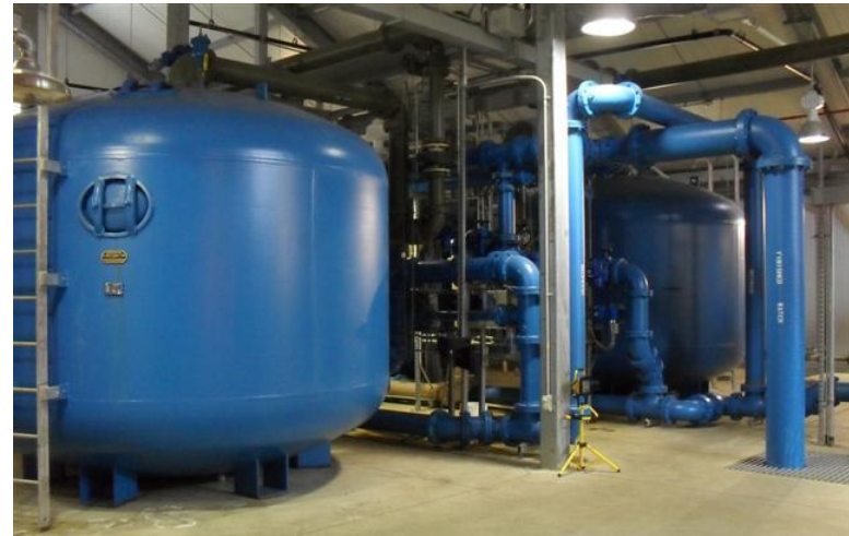
Broadway Water Treatment Plant 17
